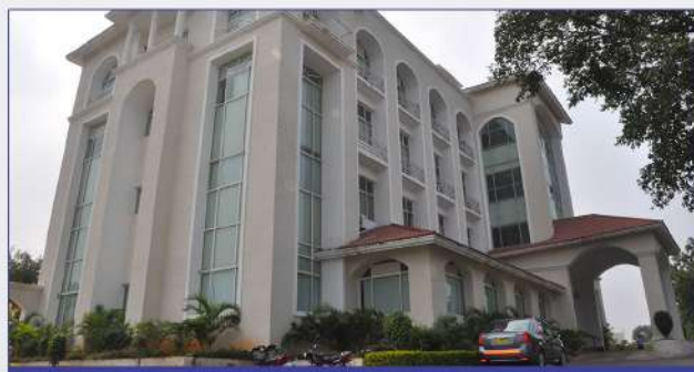
Trainees' Hostel Building (CPC Campus)
